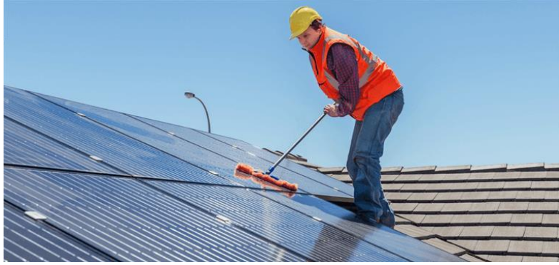
Fig 1.25: Picture of Cleaning PV panel
